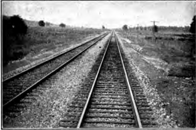
Double Track Installation Steel Cross Ties, Duquesne Rail Joints
